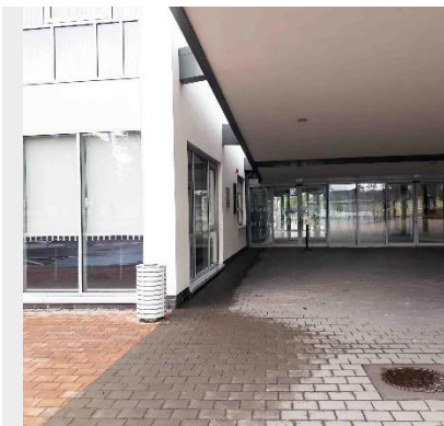
Areas at front entrance canopy
