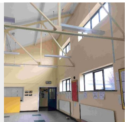
General Purpose Room glazing.
