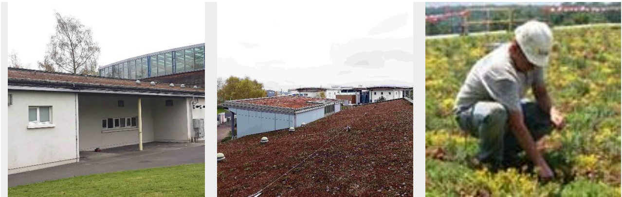
Example of single storey school with a green roof.
