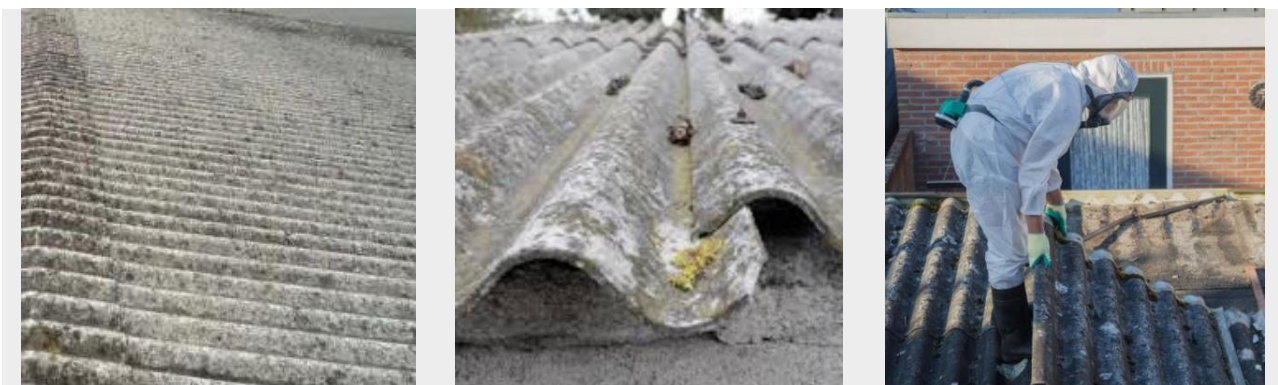
Example of asbestos roof.
