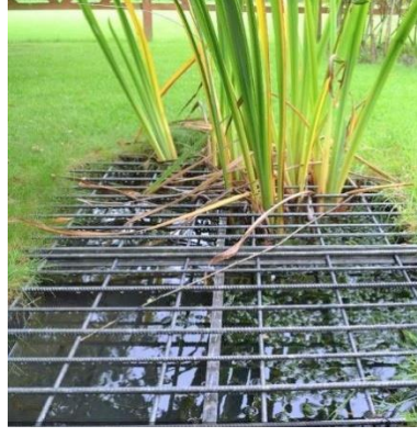
Pond with safety grid
